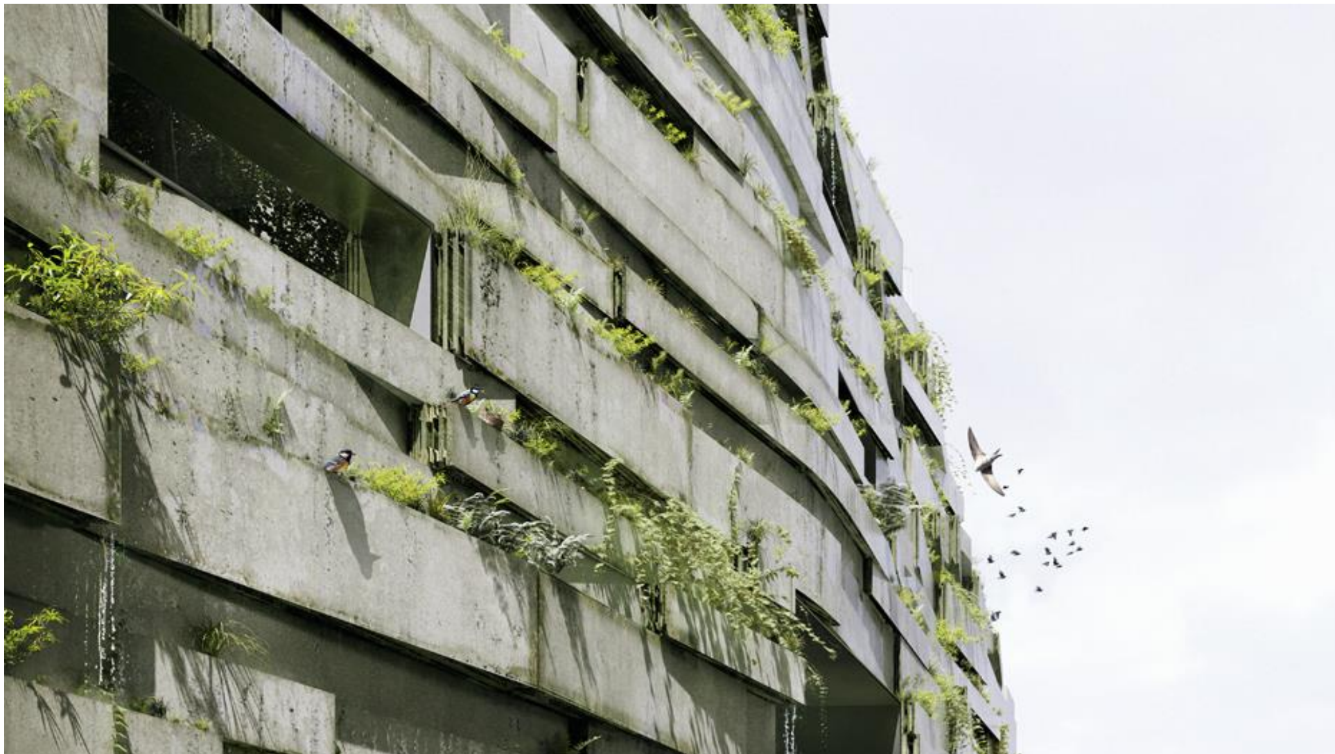
Detalle fachada vegetal, Chartier Dalix, 2014
